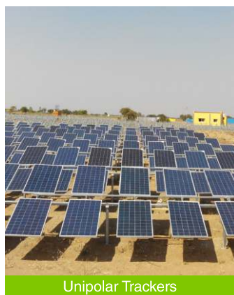
Ground Mounted Trackers
